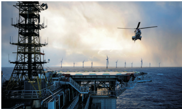
Hywind Tampen, pioneering floating offshore wind technology
